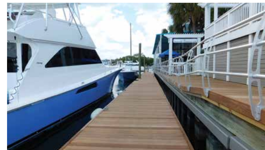
Ipe hardwood decking, timber frame.
