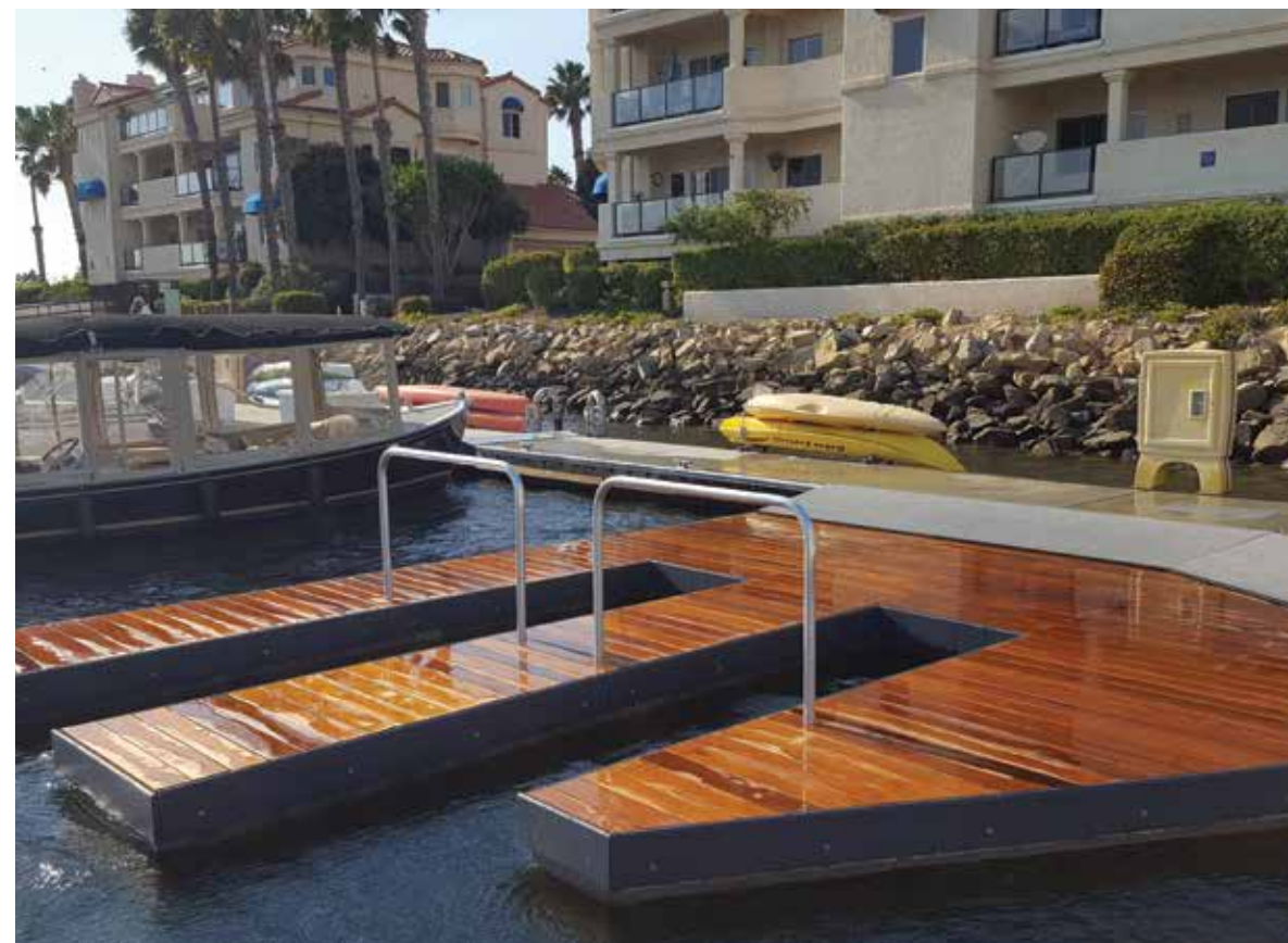
Low freeboard, concrete dock, decked in lpe
